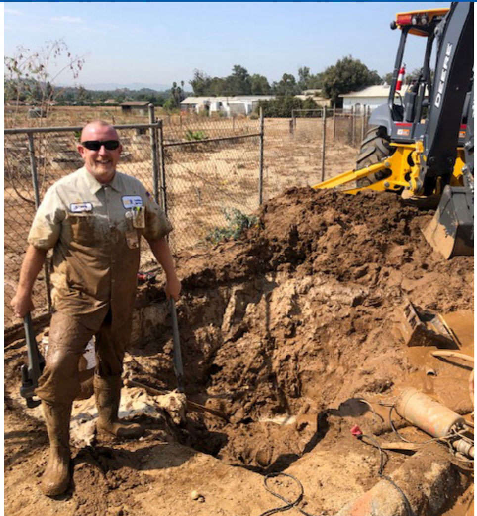
Steve Crook, lead plumber, uses a backhoe to dig out a leaking water line at Agricultural Operations, applying a clamp to stop the flooding and triaging the site. (UCR/Courtesy Steve Crook)
