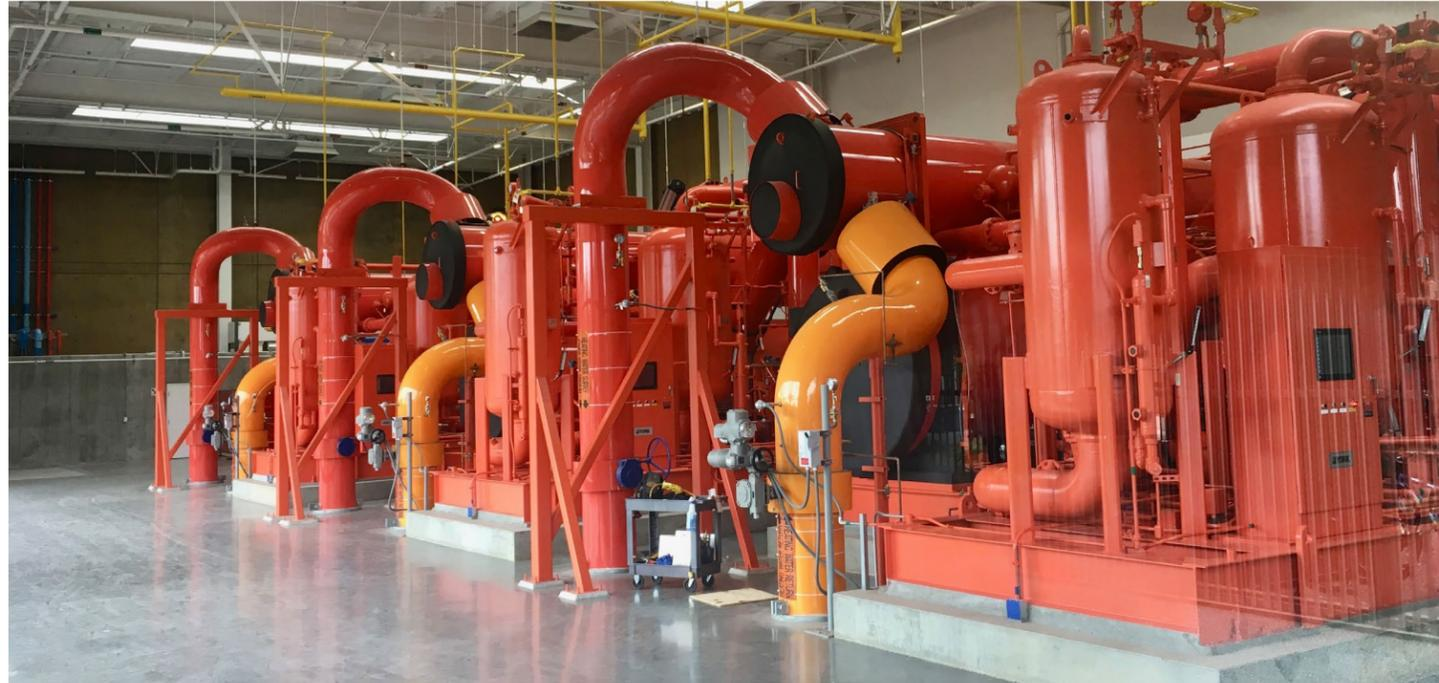
Figure 3-2: Example of WWHP Units<sup>13</sup>
