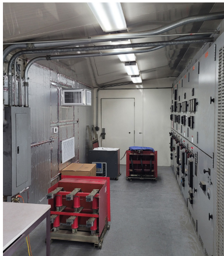
A substation HVAC project reduced peak temperatures of 130 degrees in the summer to now only upper 80s. (UCR/Bill Hensche)
