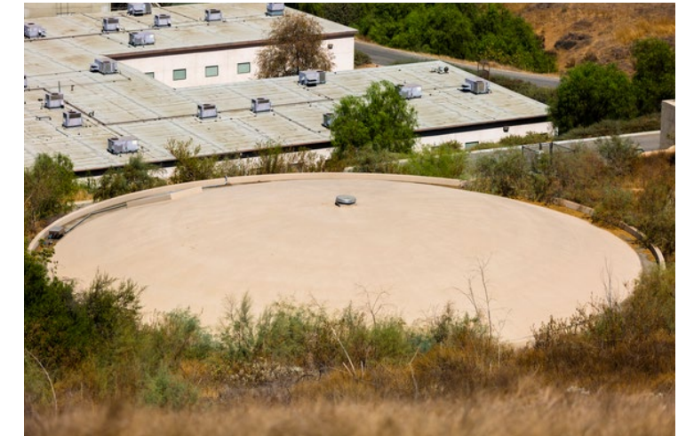
Figure 3-5: One of UCR's Three TES Tanks
